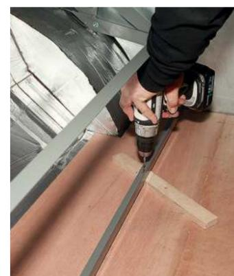
**18** Check once again that the lower support frame is straight and true. Using some offcuts of wood, lift the lower framework up slightly and slide the offcuts under so you can drill pilot holes for the self-tappers that will secure the frame to the ply floor. As per the instructions, fit one either side of the frame
